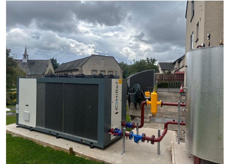
A new Air Source Heat Pump at our Castlebrae Glebe Retirement Housing + development in Edinburgh
