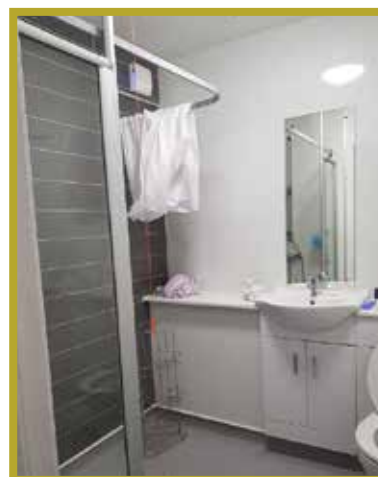
Shower room replacement
