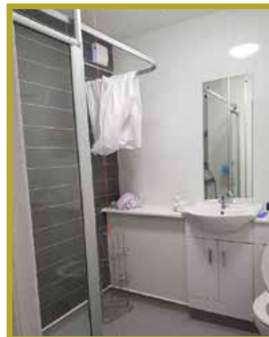
Shower room replacement
