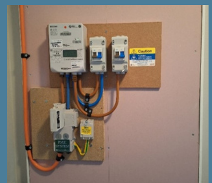
New supply cable and meter
