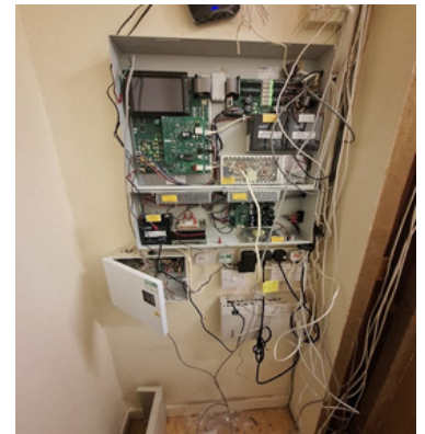
New Control Rack Being Installed
